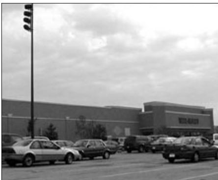
Many large parking lots sit half empty for much of the day and could easily be shared by several uses.
