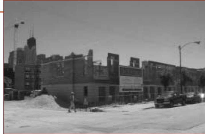
Old Town Village East under construction
