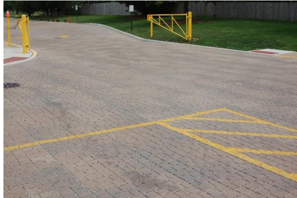
Jay Stream School Permeable Paver Parking Lot, Carol Stream (2016)
